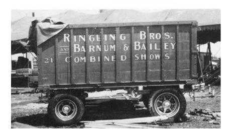
Seat Plank Wagon No. 21 was one of seven identical wagons. These photos show the wagon as it look in 1944 after having been mounted on pneumatic tires.
