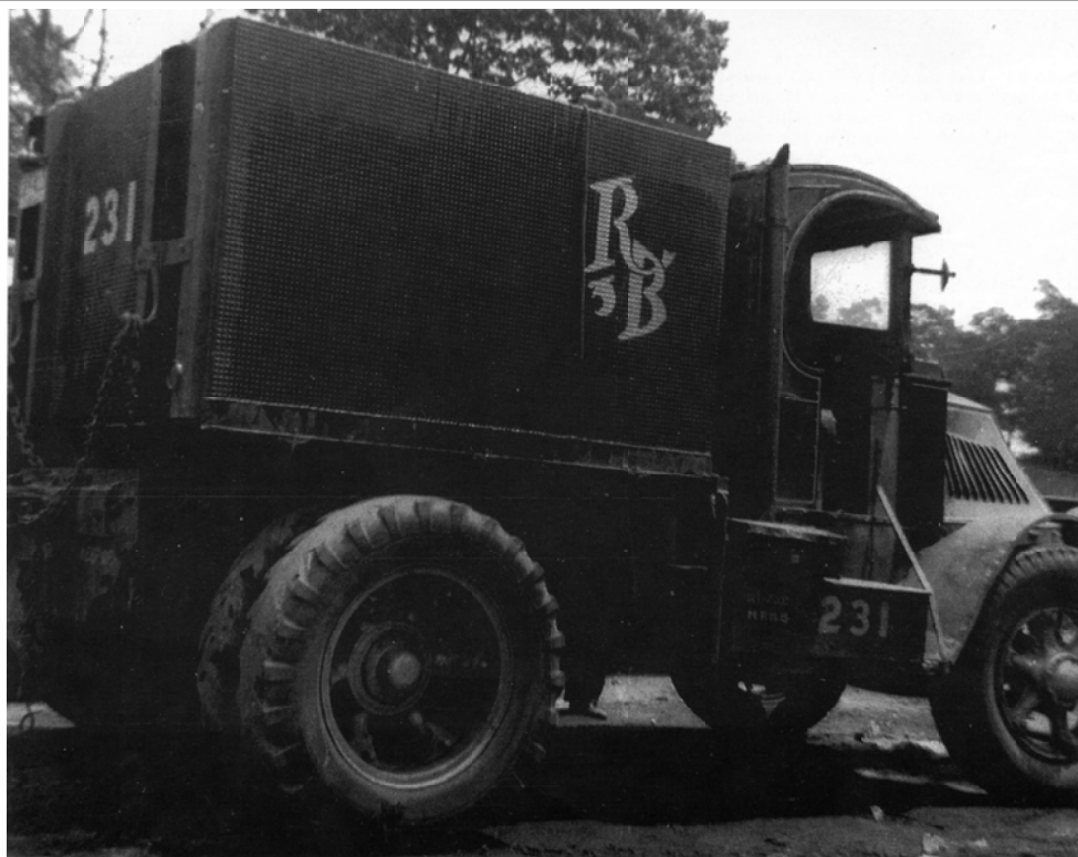
Photo 5 - RBBB No 231 with a large, high , all steel water tank. Note the exhaust stack for the diesel engine and exterior support strap on the running board to support the extra tool box. [Dyre Reynolds Photo]
