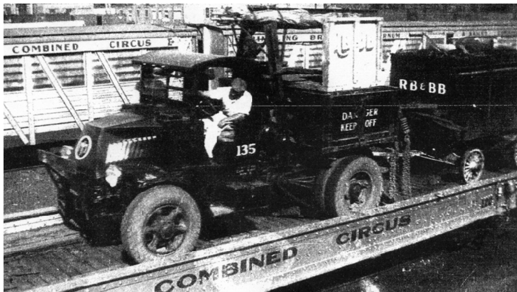
Photo 10 - RBBB No. 135 pulling a wagon over flats in 1936. Note the Gilly wagon riding on top of storage area and hard rubber tires replaced by pneumatic ones. [Conover Collection]
