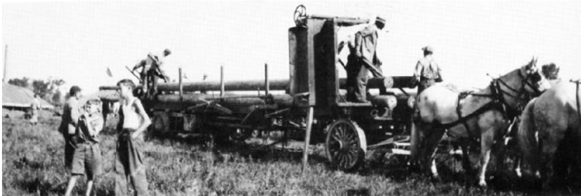
Photo 2 - Unloading big top center poles from pole wagon on RBBB in 1932. Note how the front of the wagon is tipped over to allow the center poles to be rolled off the wagon. [Carver Collection]
