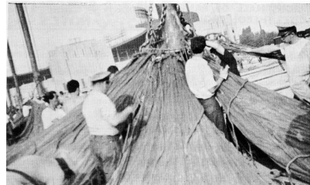
Sections being laced to the Bale 'Ring' - Note how the lacing loops on canvas sections hang from canvas. These get laced through eyelets in next section. then through the next loop and so on down the sections, thus lacing both sections together making a zipper effect, and tied at the outer edge to keep the lace from coming open. [A Templeton photo]
