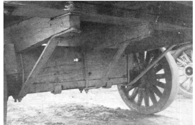
Photo No. 13 – Back view of rear undergear
